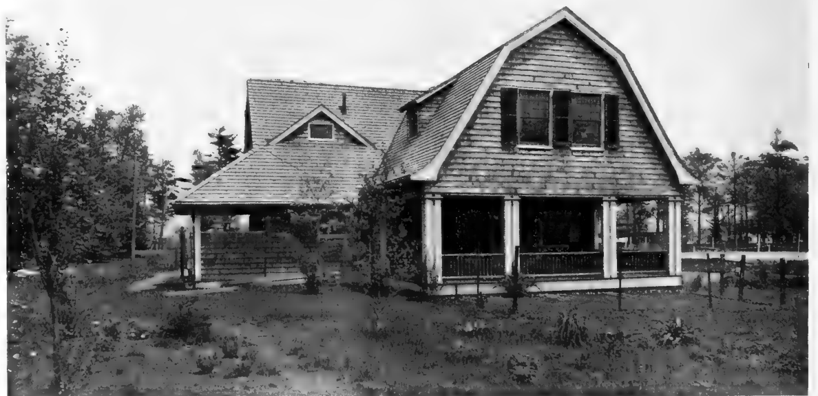
12—A Feature of the Exterior is the Long Gambrel Roof, and the Piazza, which in Winter is Inclosed with Glass
